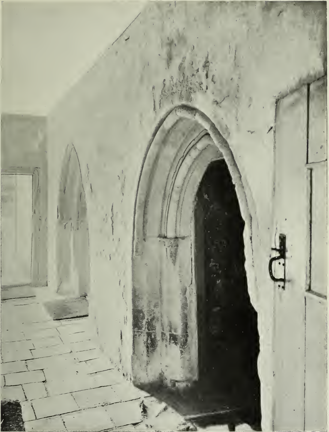
LITTLE CHESTERFORD: THE MANOR HOUSE. Doorways to Screens-passage ; early 13th-century.
